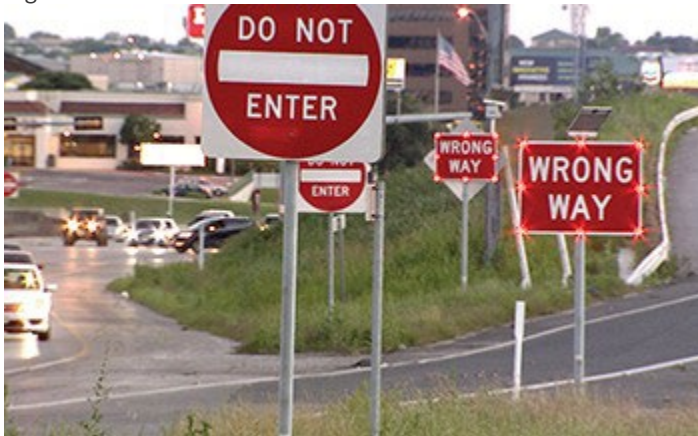
The project showed that flashing LED Wrong Way signs reduced the number of wrong-way driving incidents.
